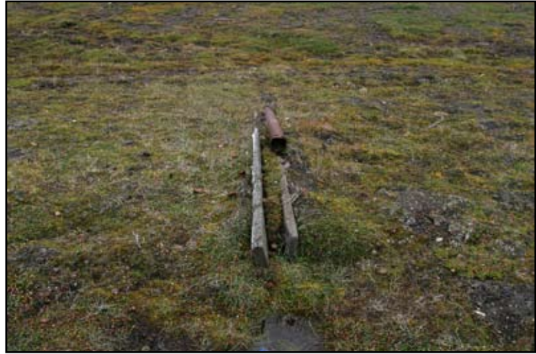
Fig. 4.15 Drain pipe and wood enclosure in roadbed. Photo by Larry Mishkar/MTU.
