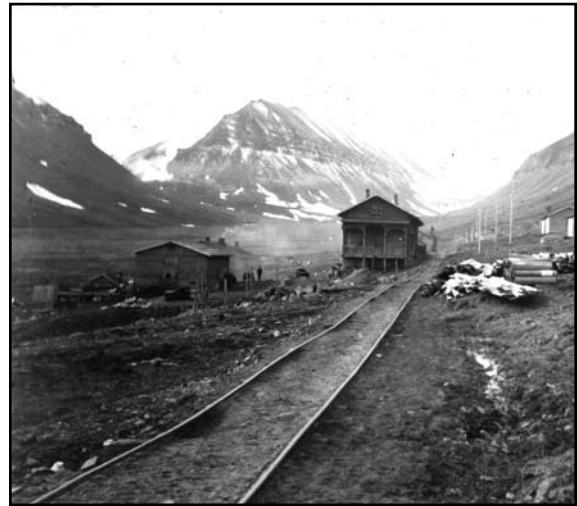
Fig. 4.13 Undated photograph showing 3-foot gauge railway. Michigan Technological University Archives and Copper Country Historical Collections.
